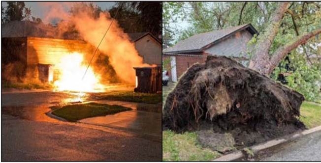
Figure 1: Downed powerlines and felled trees pose a significant risk during storm season. Images from a recent storm this season.
