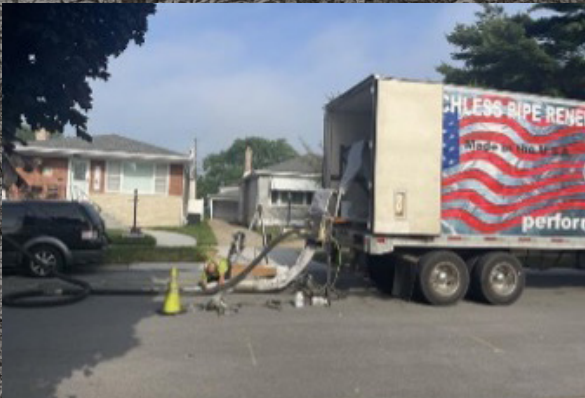
Buffalo Ave Sewer Lining
