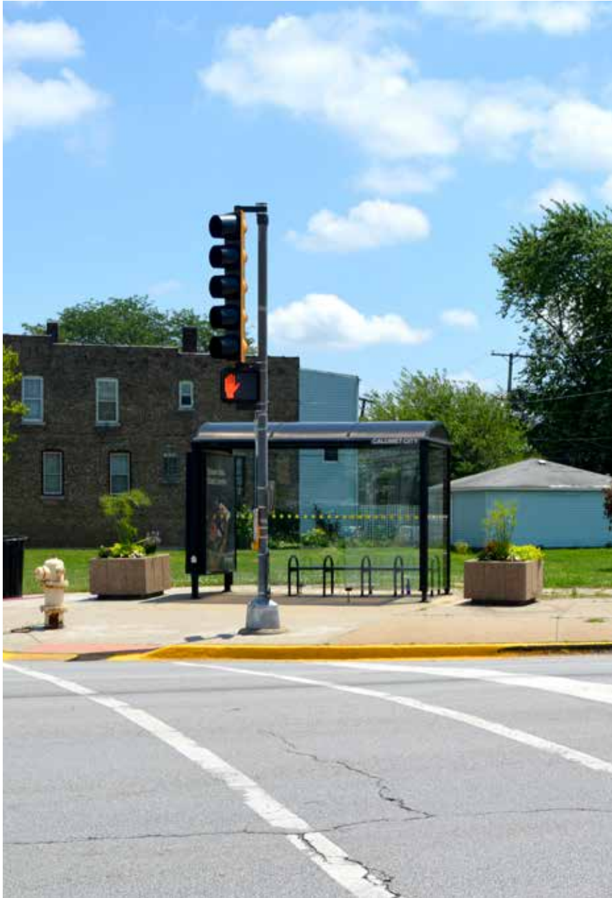
Photo 6: PACE Suburban Bus stop shelter at Pulaski Road and Burnham Avenue Source: Great Cities Institute
