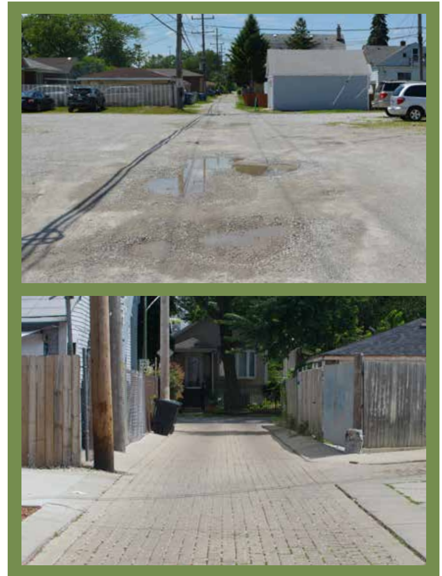
Figure 15: Top - Existing alley behind Burnham Avenue businesses. Bottom - Alley with permeable brick paving in Chicago. This treatment reduces flooding by allowing water to percolate into the ground below, rather than run-off to storm water drains. Source: Center for Neighborhood Technology
